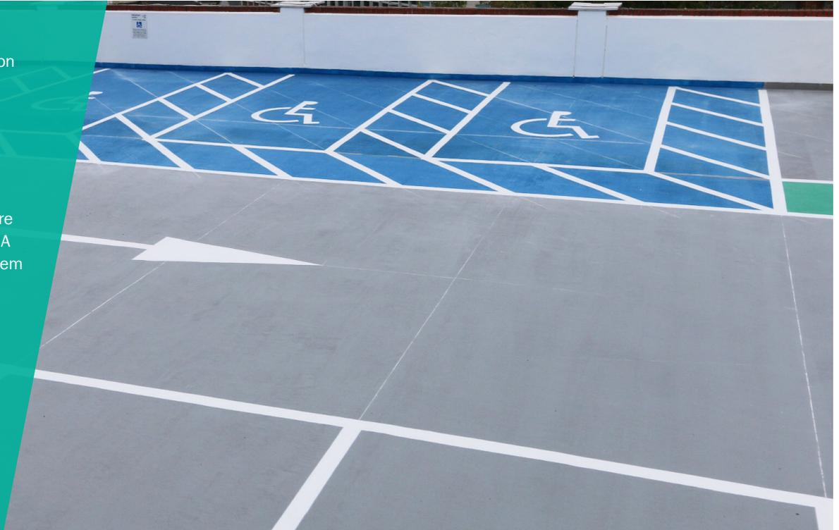
**The Rose Car Park required modernisation and TREMCO's MMA system was specified for both the internal deck and external deck. The system which has ETAG accreditation is particularly well suited to projects that require a rapid turnaround as it has a cure time of just 30 minutes and a walk on time of 1 hour.**
